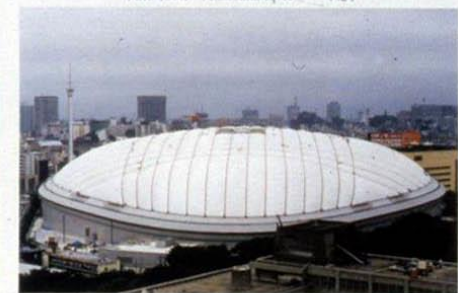
8.30 a.m. Internal pressure reaches 30mmAq and roof is fully inflated.
