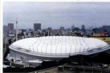
6.25 a.m. Internal pressure reaches 14.5mmAq
