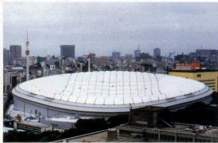
6.10 a.m. Internal pressure reaches 13.5mmAq
