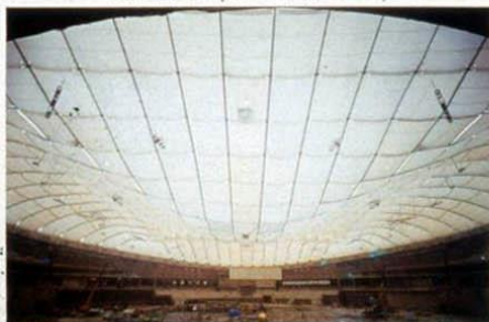
6.10 a.m. Internal pressure reaches 13.5mmAq
