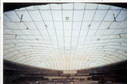
6.25 a.m. Internal pressure reaches 14.5mmAq
